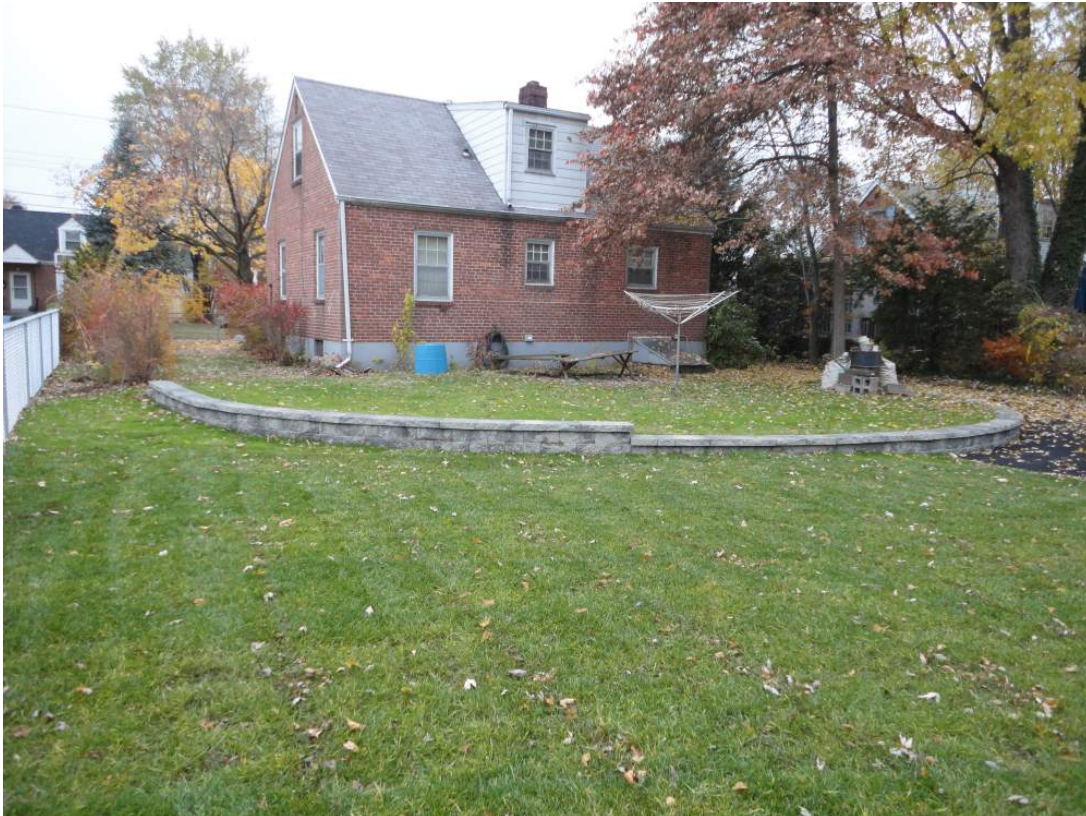
View looking northeast of fully restored back yard.
