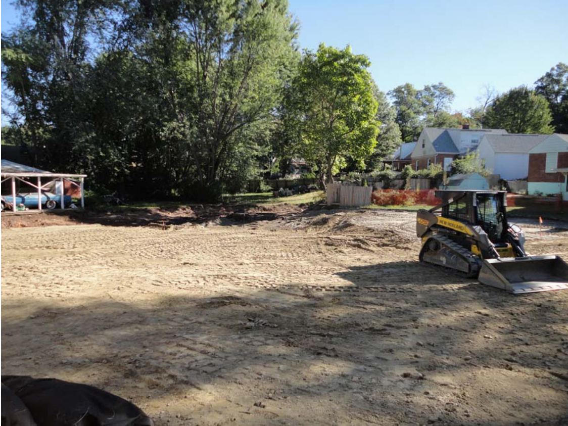
View looking northeast of backfilled back yard.
