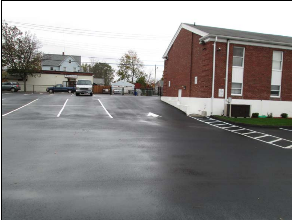
View looking west at parking area.
