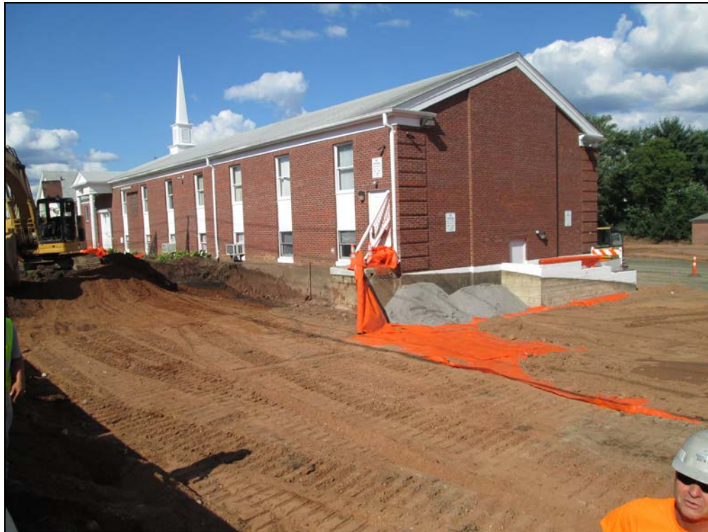
View looking northeast at excavation in front yard and parking area.
