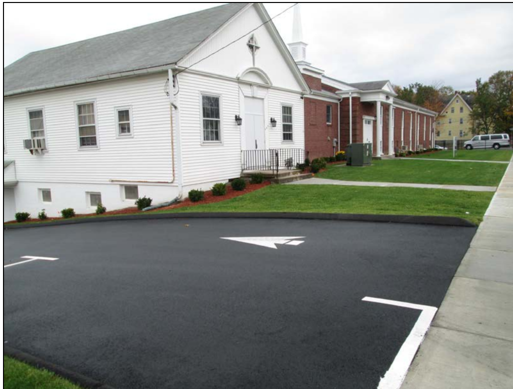
View looking southeast at restored front yard and driveway area.
