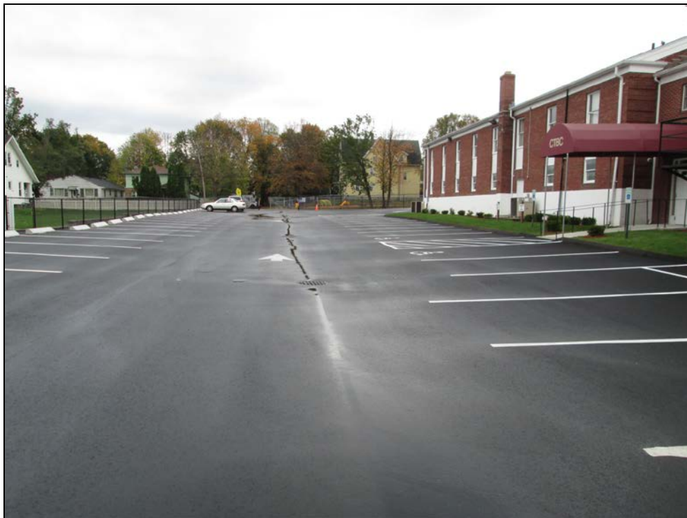
View looking south at restored back parking area.
