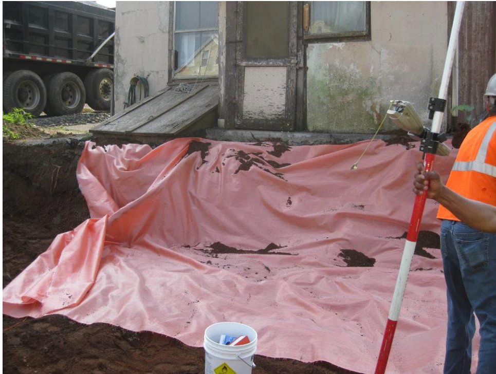
View looking West at excavated back yard
