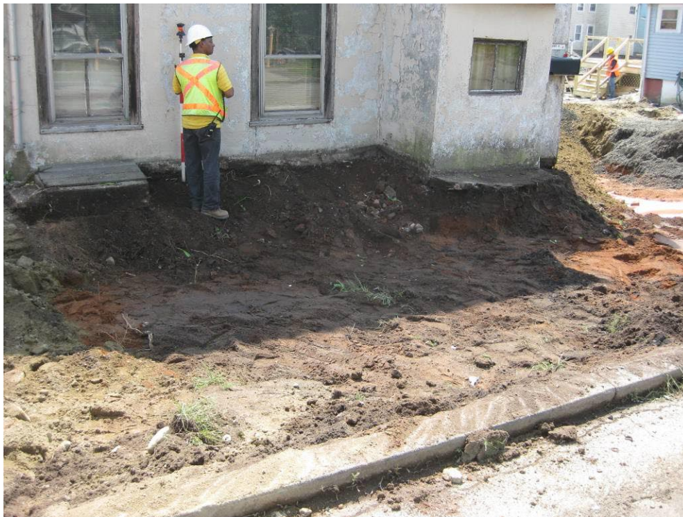
View looking Southwest at excavated front yard
