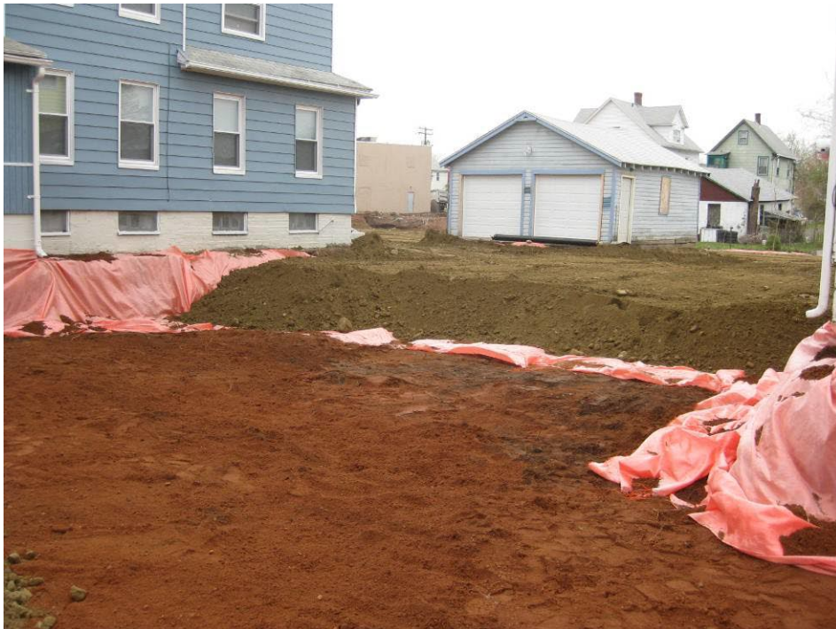
View looking Northeast at partially backfilled driveway and yard
