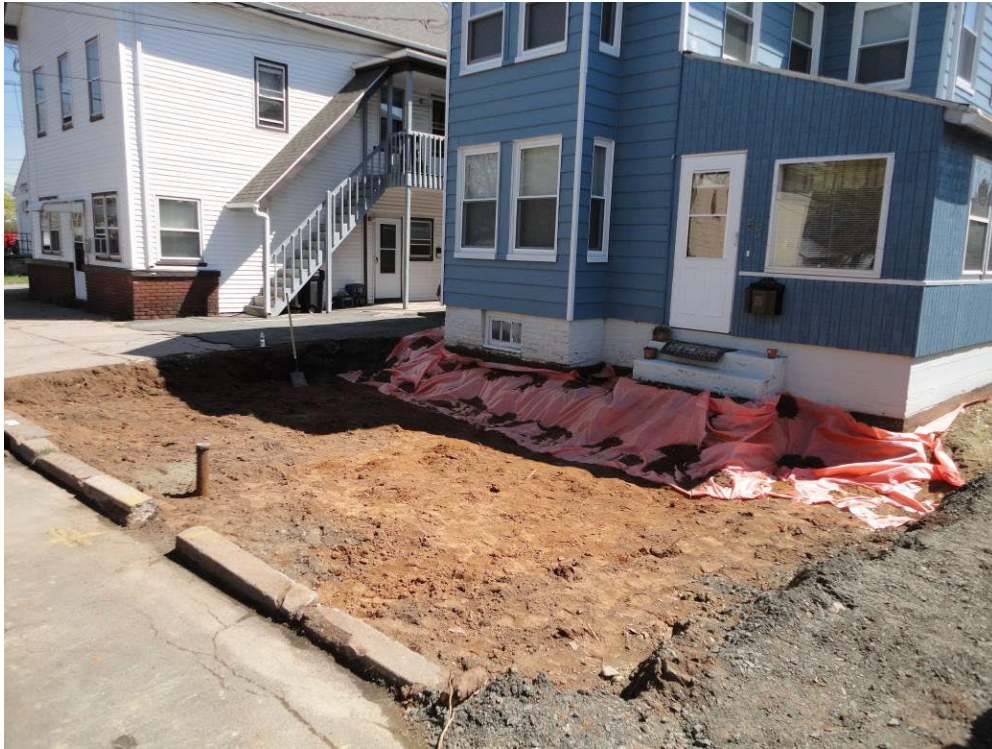
View looking Northeast at excavation area following placement of marker barrier
