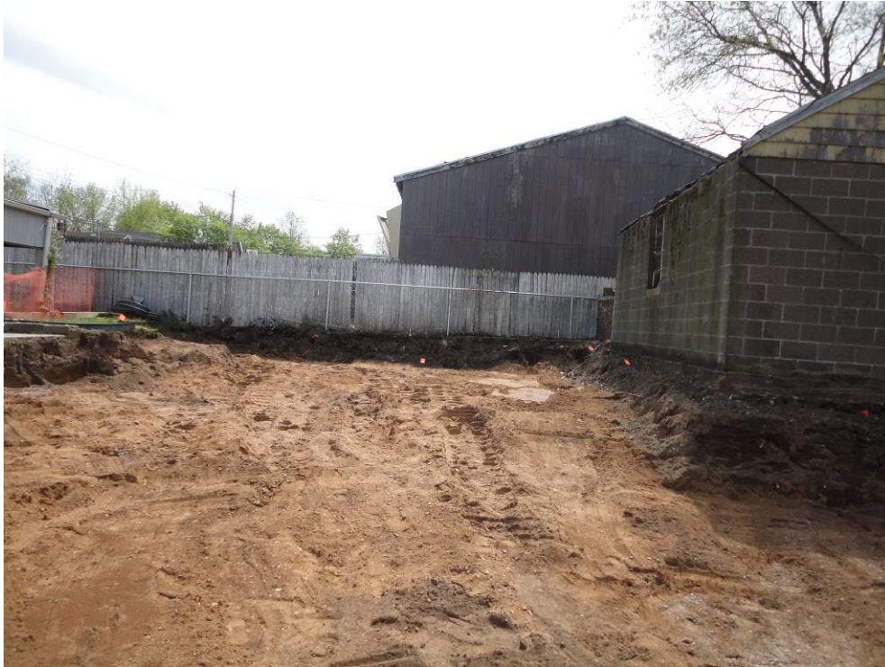
View looking South at excavated back yard
