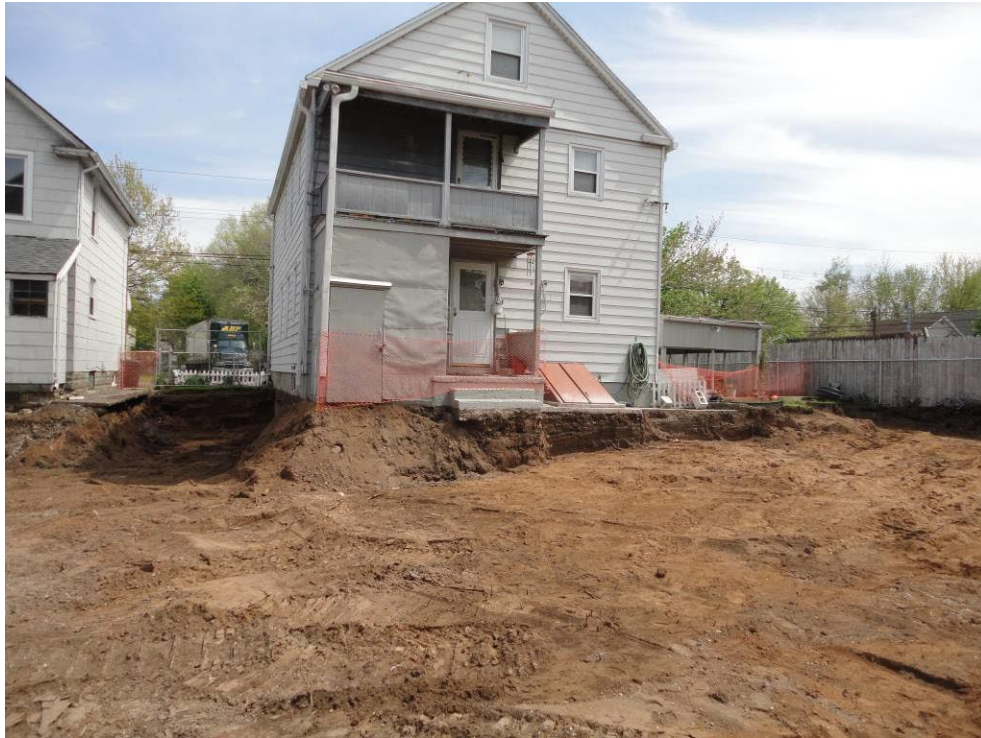
View looking East at excavation area in back yard
