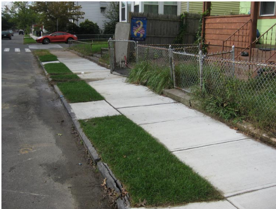
View looking South at restored sidewalk
