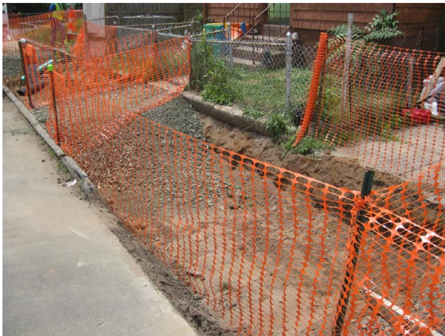
View looking South at excavated sidewalk
