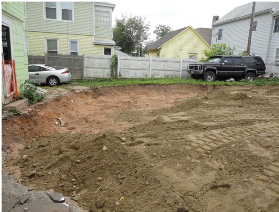
View looking South at excavated back yard
