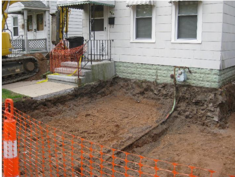
View looking Southwest at excavated front yard with utility line exposed
