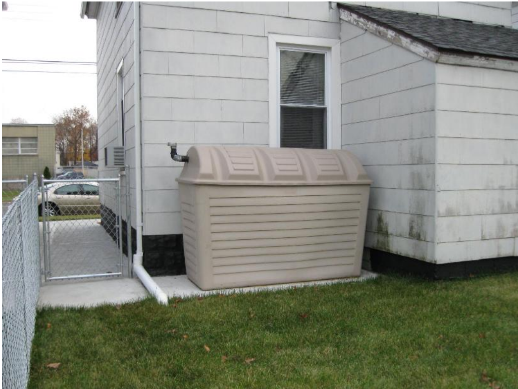
View looking east at newly installed aboveground fuel oil storage tank
