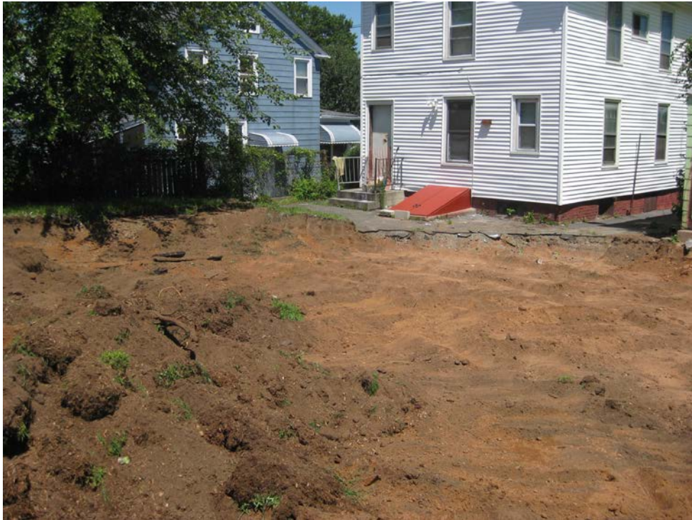
View looking Northeast at excavated back yard
