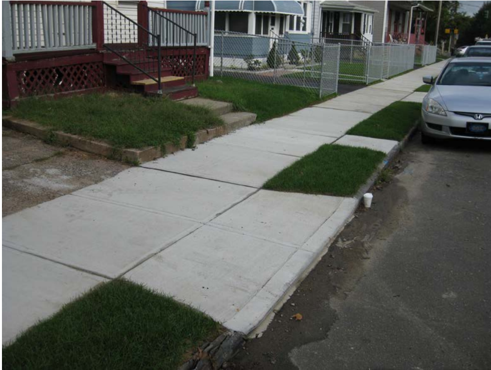
View looking Northwest at restored sidewalk
