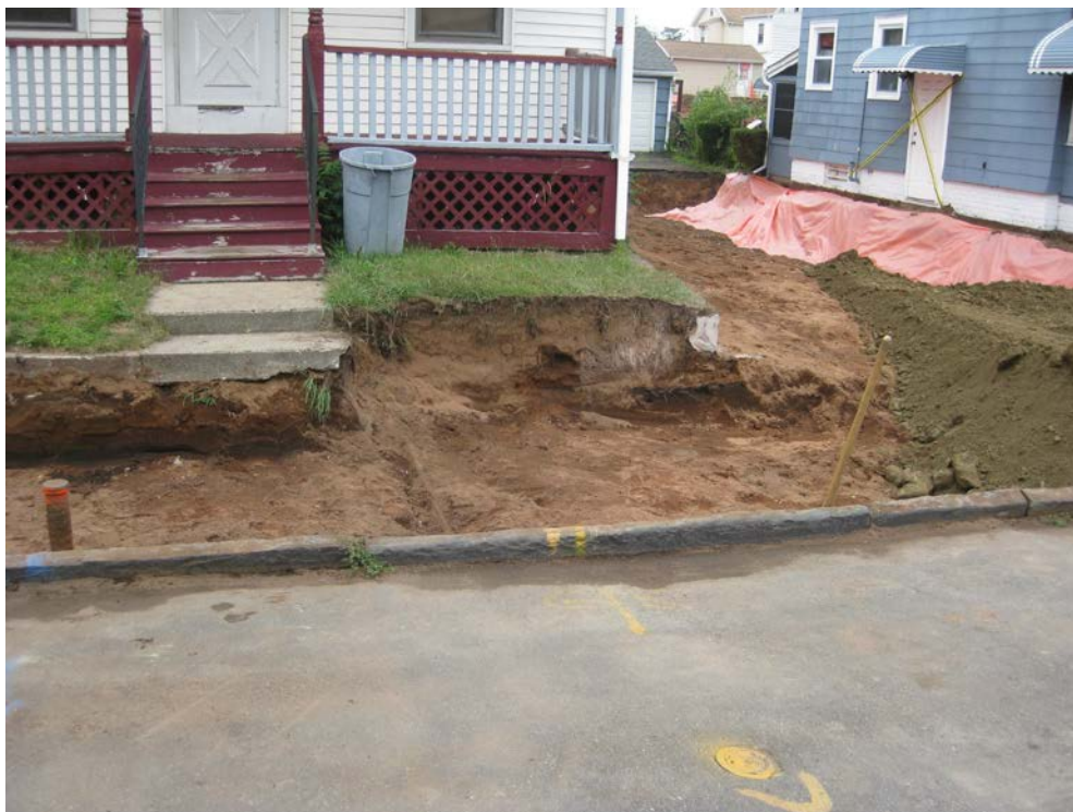
View looking West at excavated front of property
