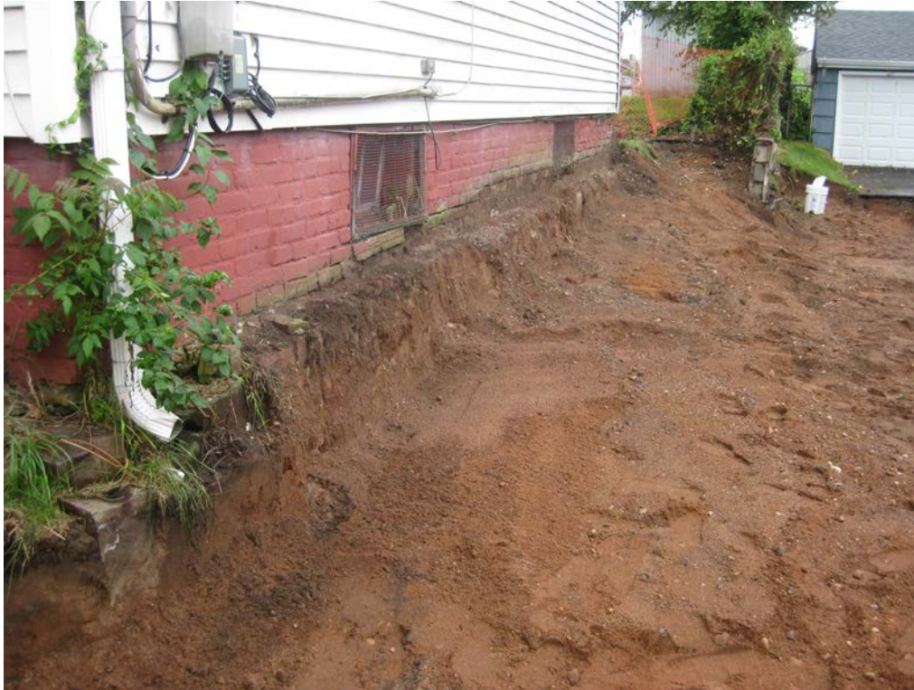
View looking East at excavated side yard
