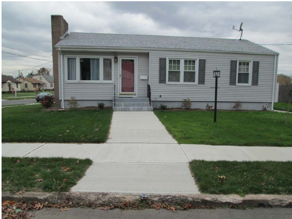
View looking west during the Fall 2012 inspection.
