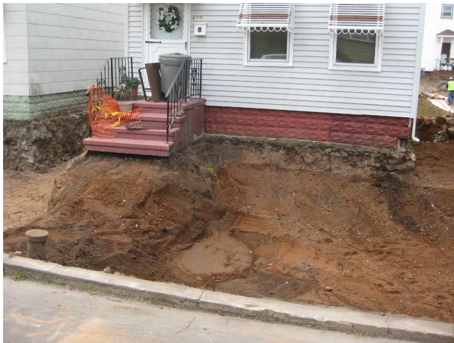
View looking West at excavated front yard
