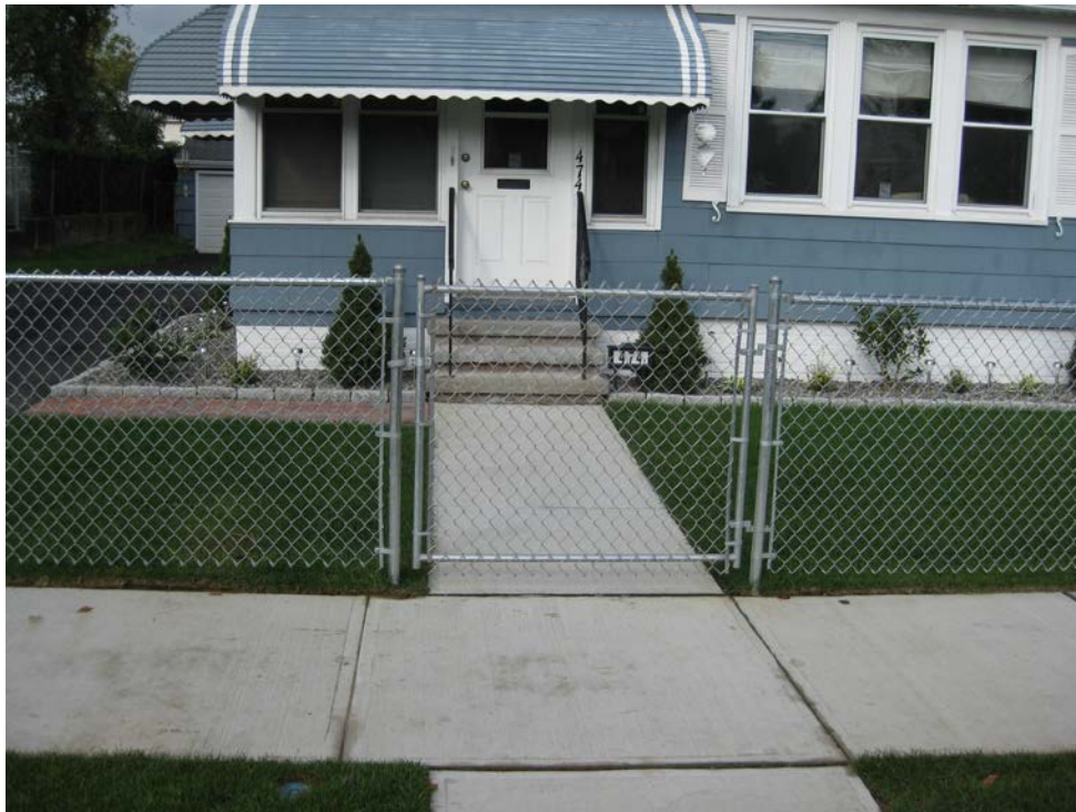
View looking West at restored front of property
