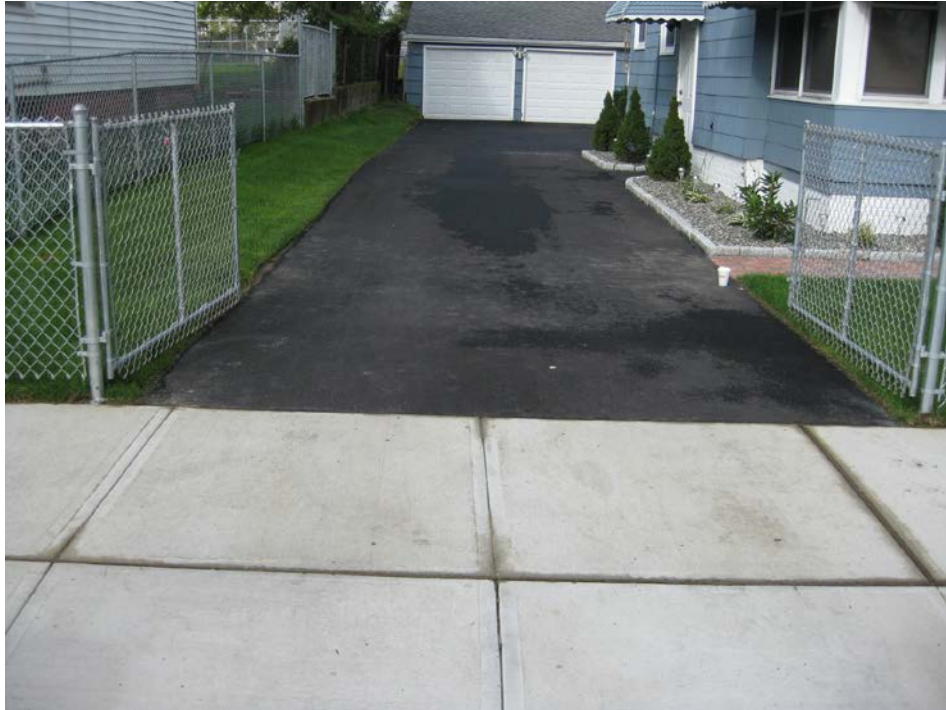
View looking West at restored driveway
