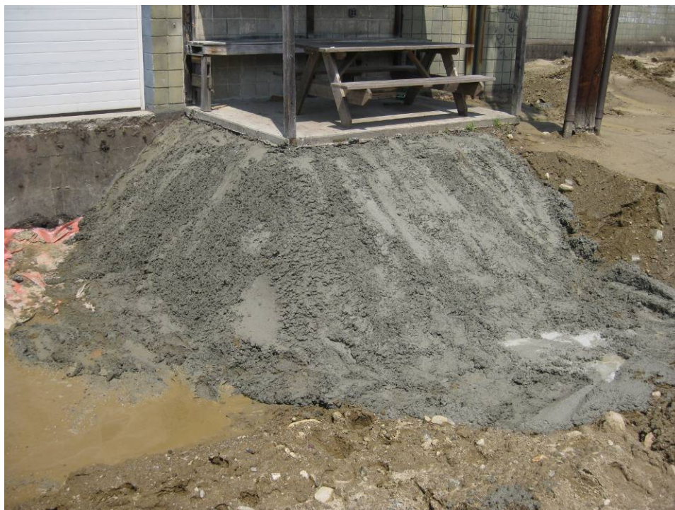
View looking West at concrete marker barrier placed near loading dock
