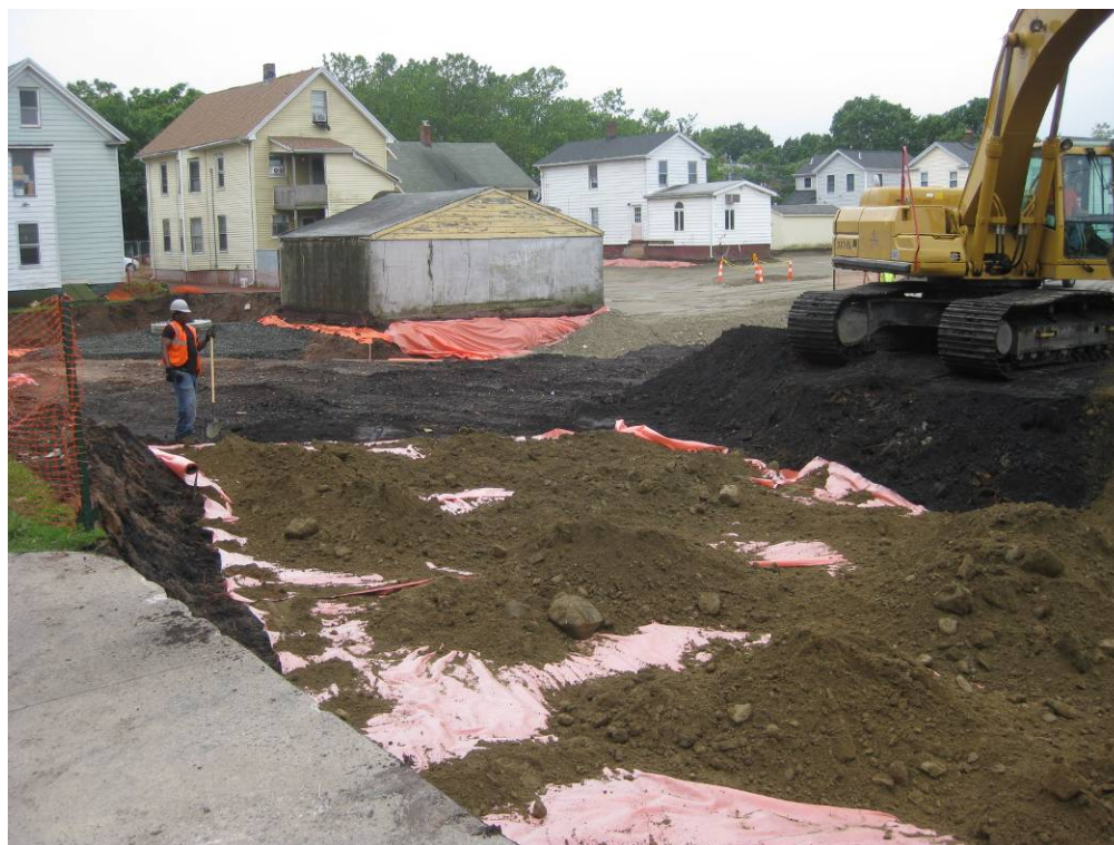
View looking Southwest at excavated Eastern edge of property
