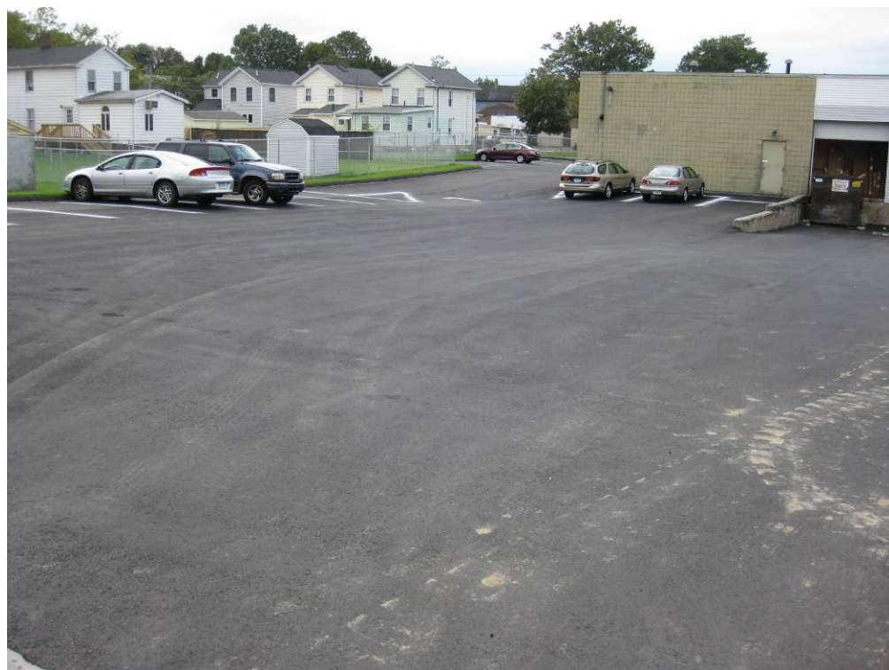
View looking West at restored parking area
