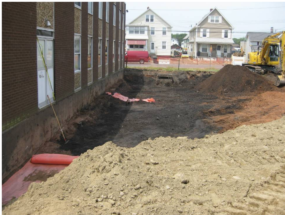
View looking West at excavation along Northern side of property
