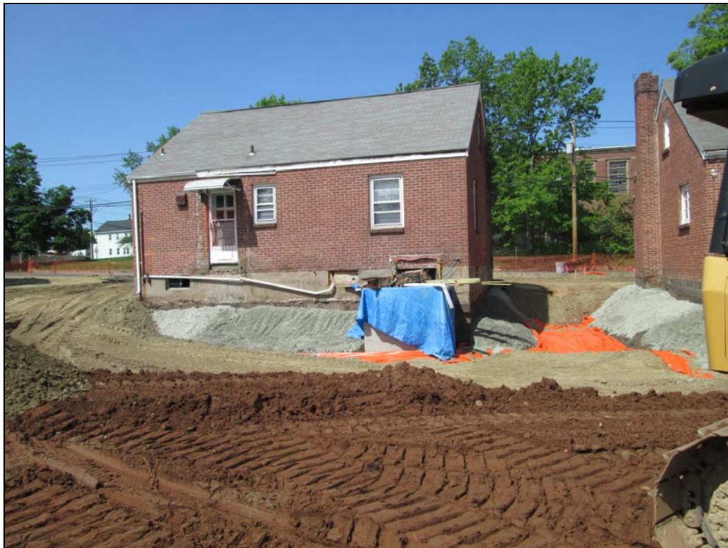
View looking west at partially backfilled back yard.
