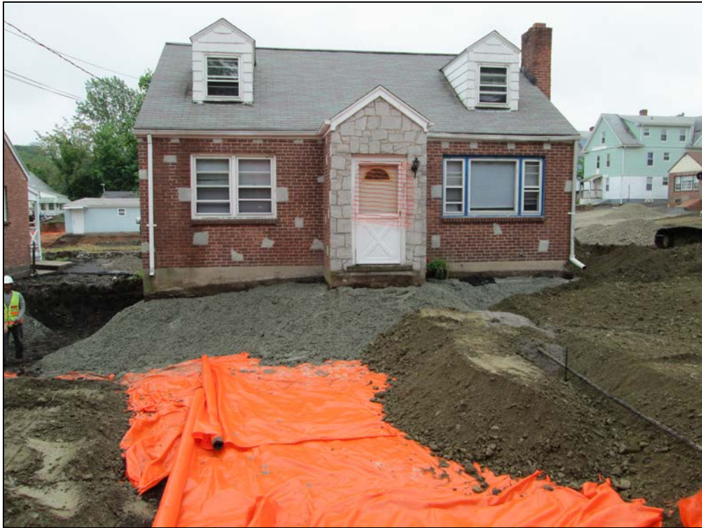
View looking east at partially backfilled front yard.
