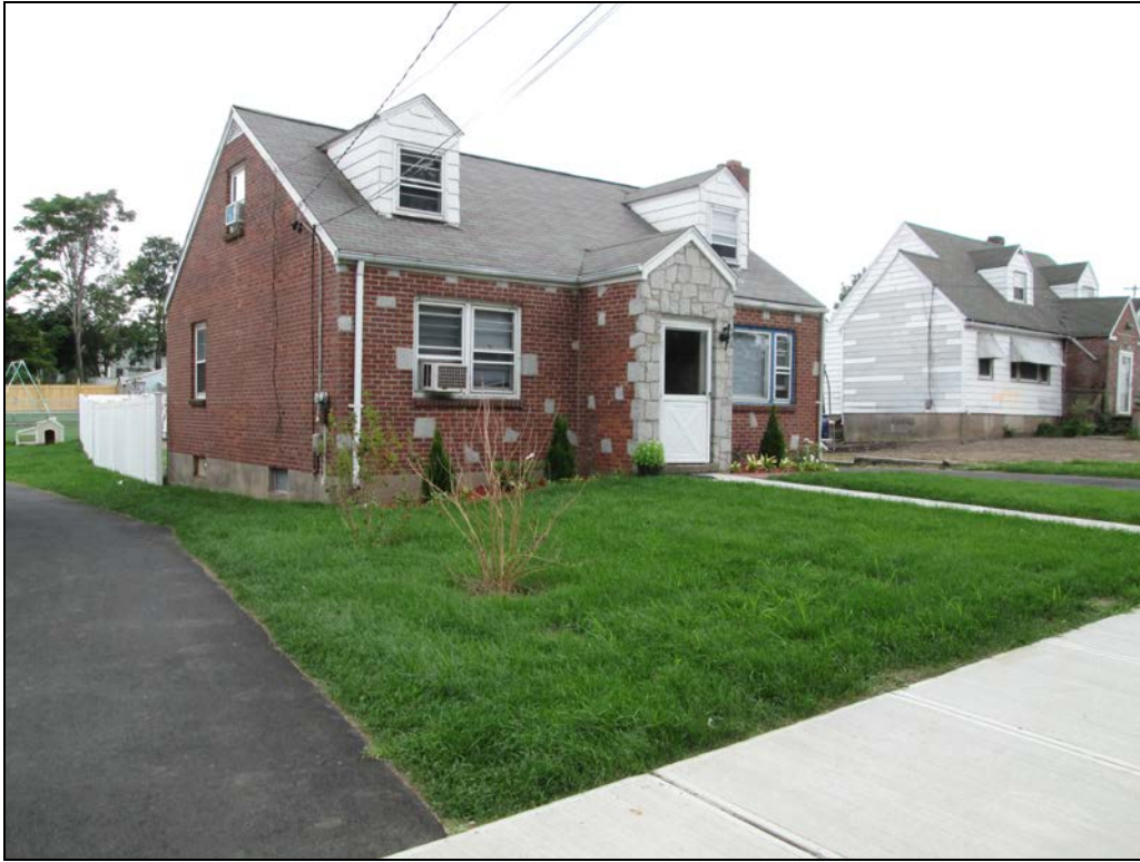
View looking southeast at restored front yard.
