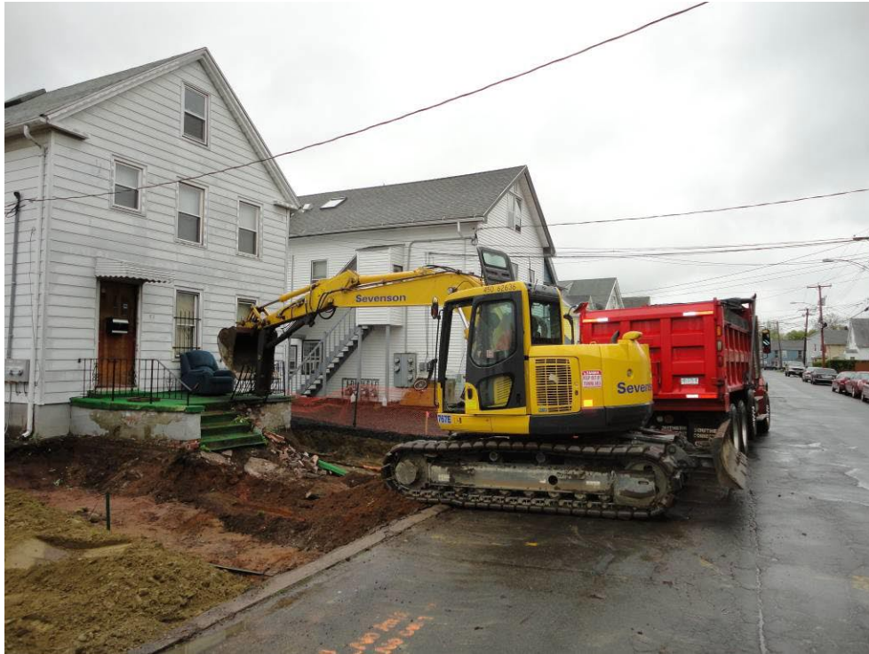
View looking South at excavation of front yard
