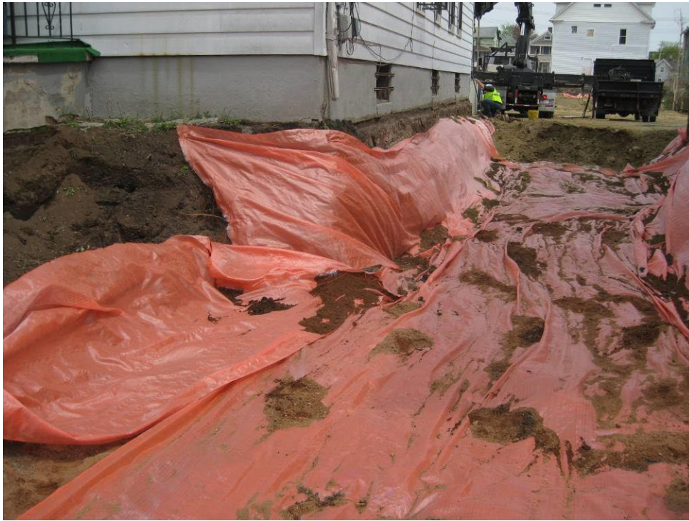
View looking East at excavation area following placement of marker barrier
