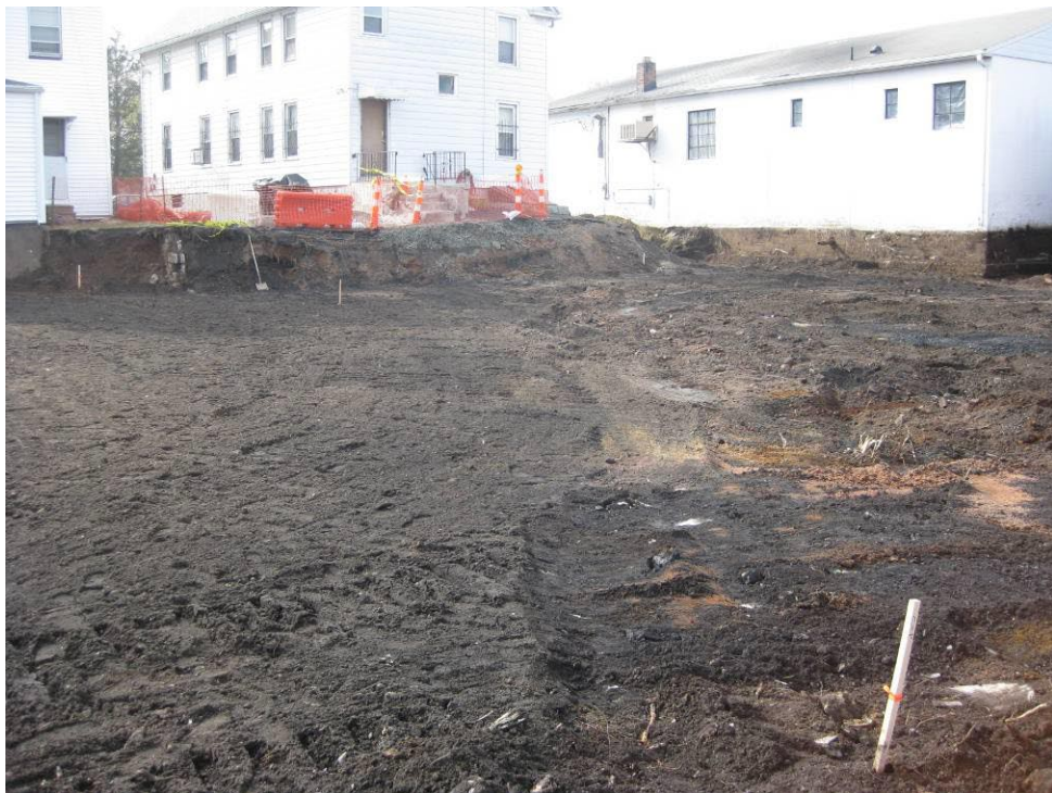
View looking Northwest at excavation area in backyard
