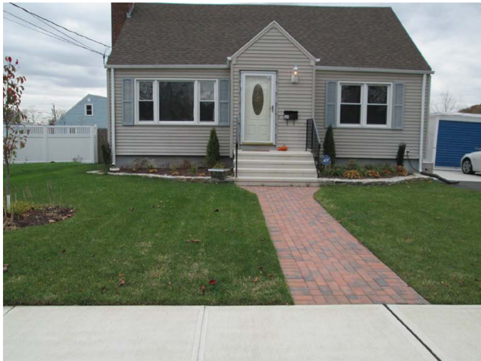
View looking west during the Fall 2012 inspection.
