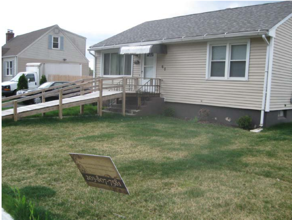
View looking southwest during the Spring 2012 inspection.
