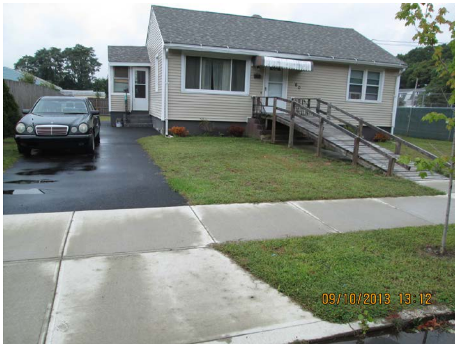
View looking west during the Fall 2013 inspection.
