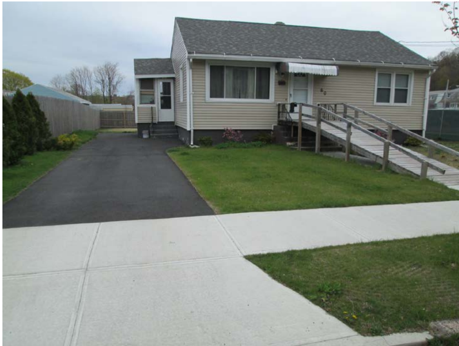
View looking west during the Spring 2013 inspection.
