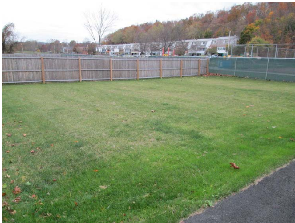
View looking northwest during the Fall 2012 inspection.
