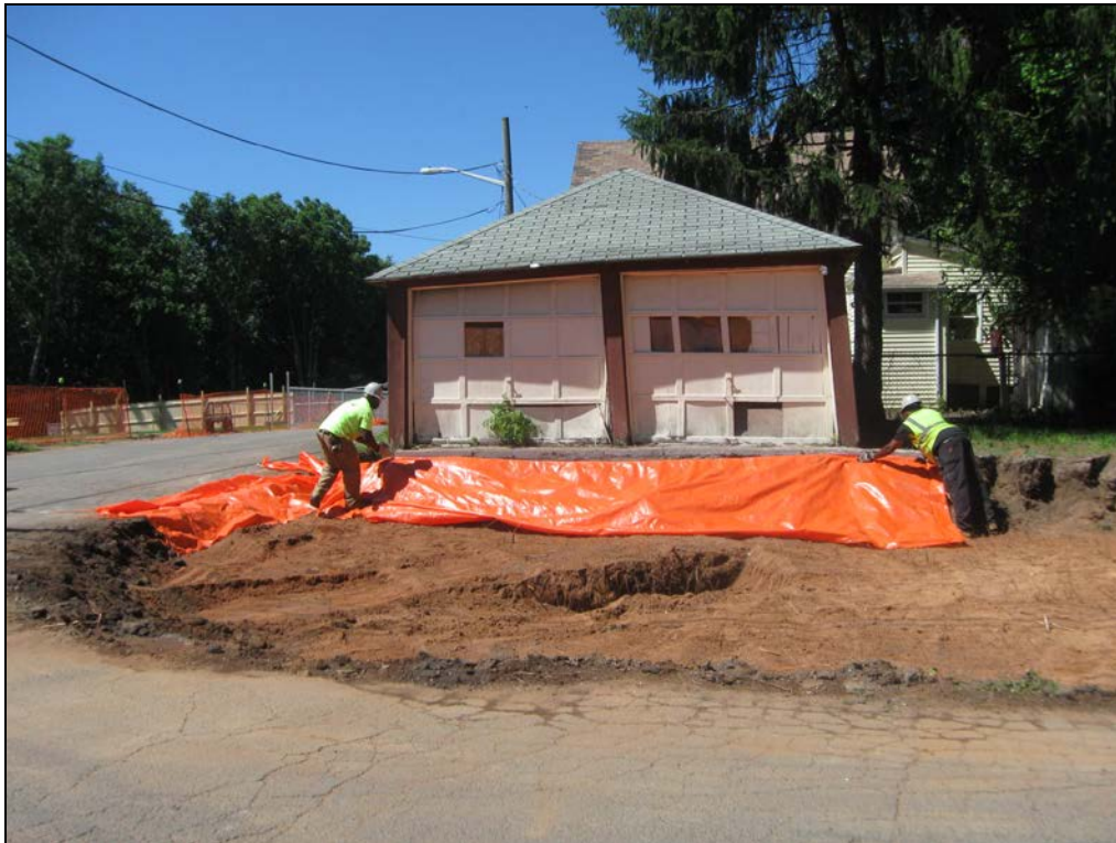
View looking northeast at marker barrier being installed.
