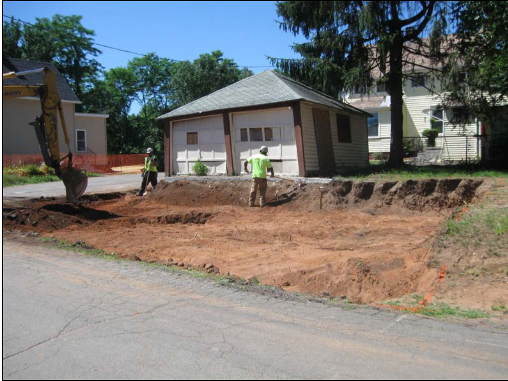
View looking northwest at excavated yard.
