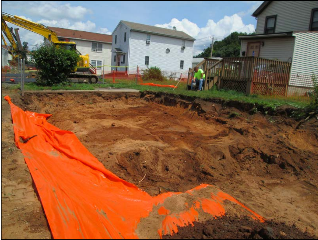
View looking northeast at excavation along Remington Street.
