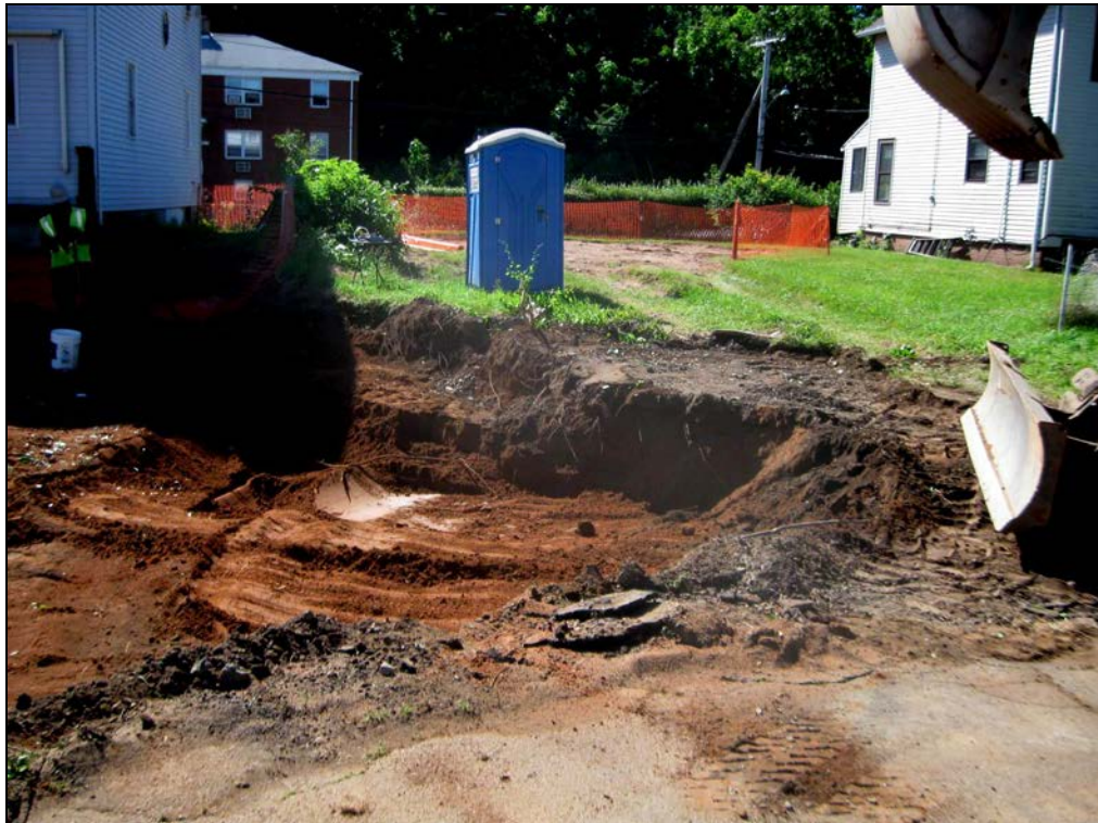
View looking east at excavation along northern boundary of property.
