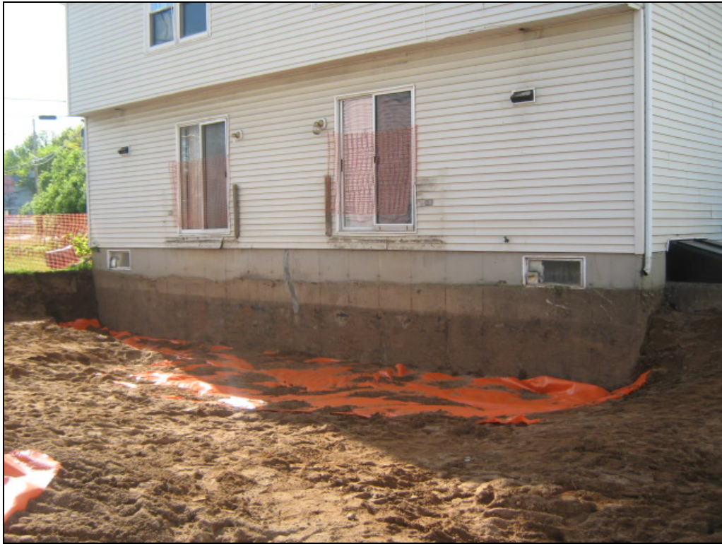
View looking southeast at excavated side yard.
