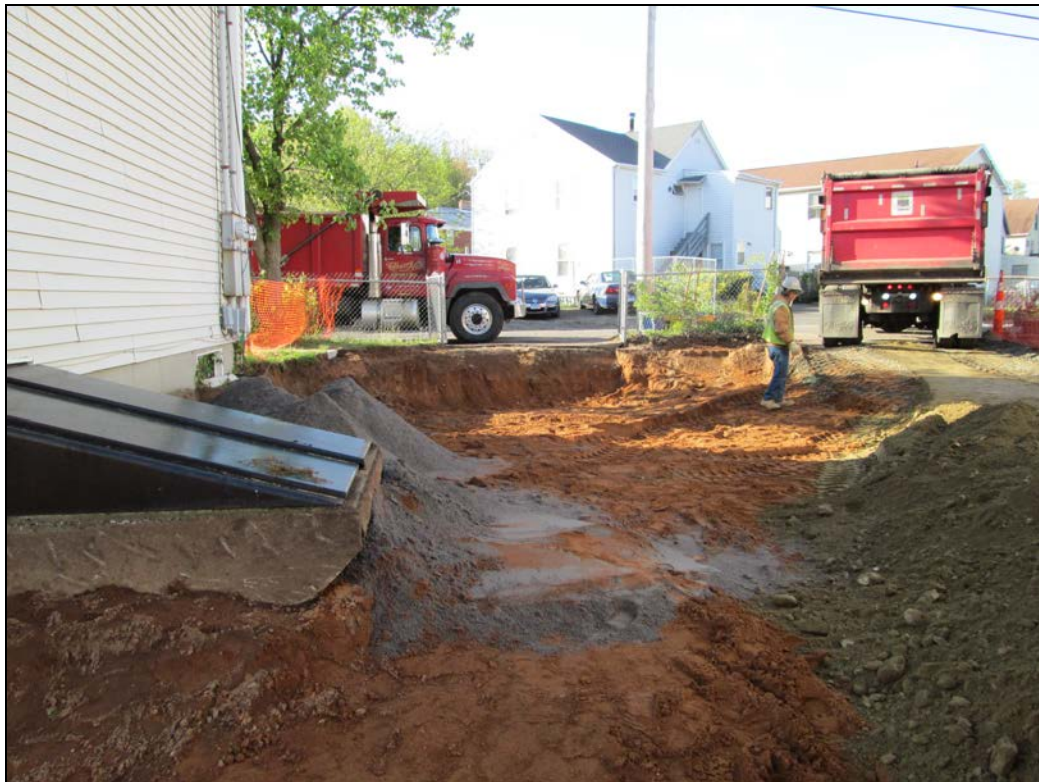
View looking south at excavated driveway area
