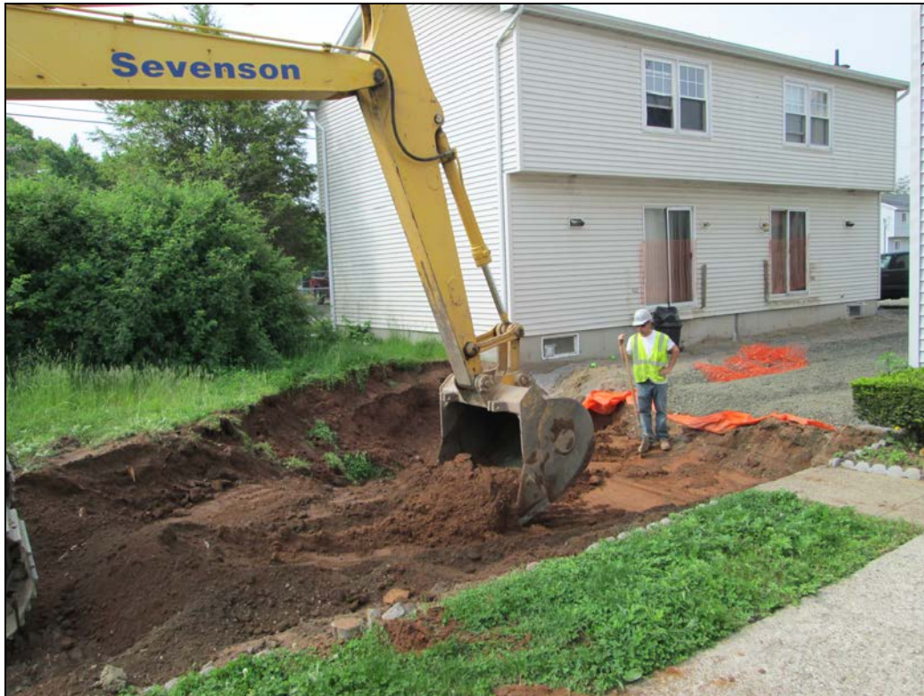
View looking southwest at excavation activities in side yard.
