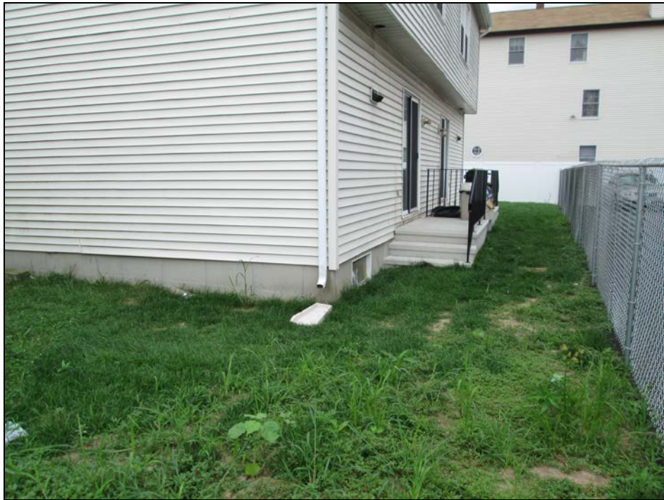
View looking west at restored back yard.
