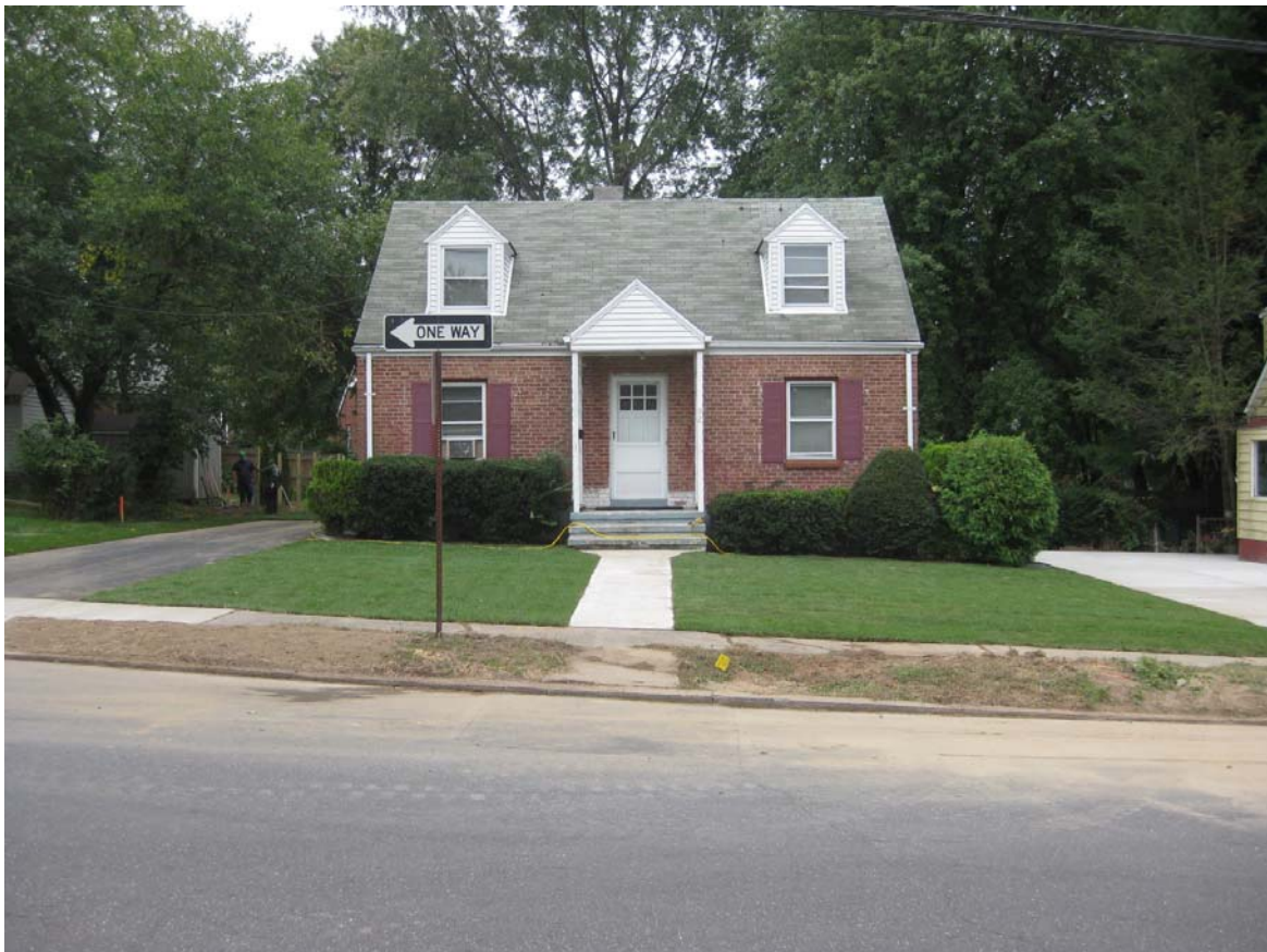
Looking south from across Morse Street at full restored property.
