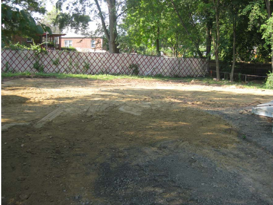
View looking south at backfilled back yard.
