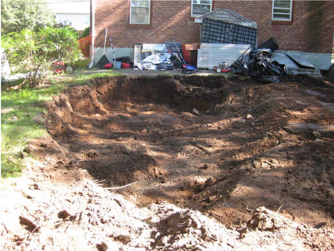
View looking north of excavation in back yard.
