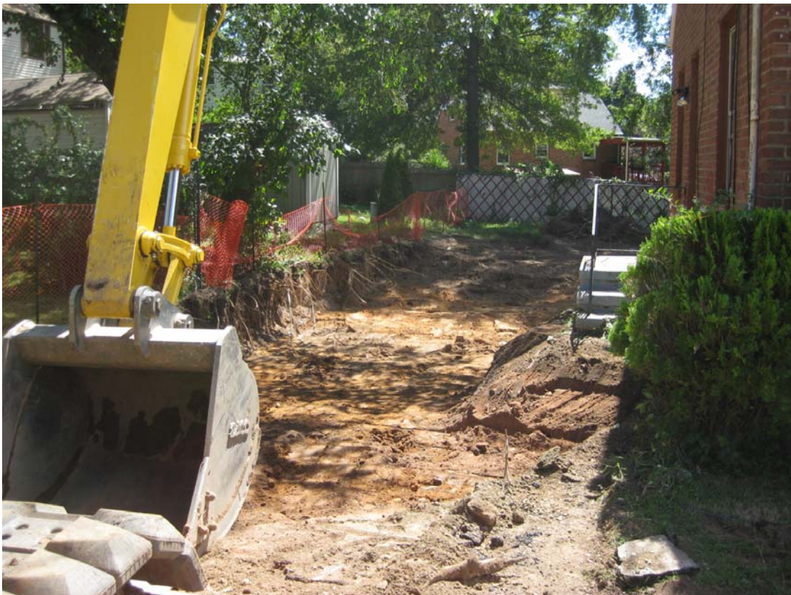
View looking south at excavation of driveway area.
