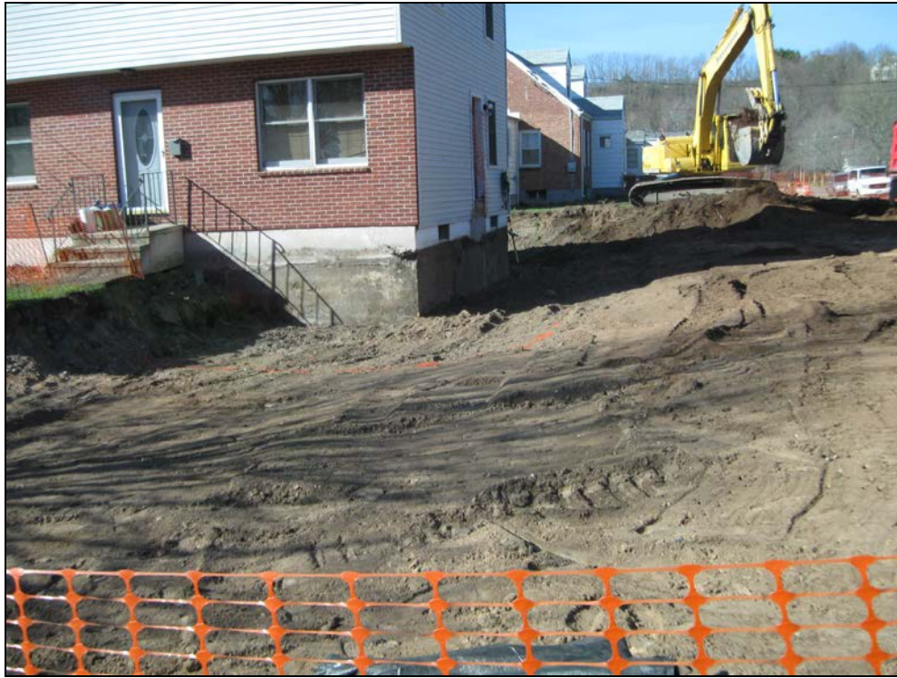
View looking north at excavated front and side yard.
