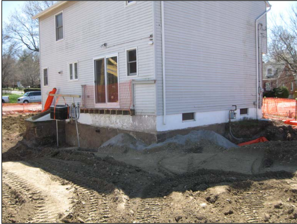
View looking southeast at excavated back yard.
