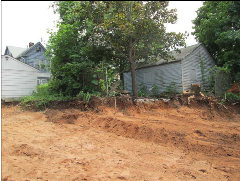
View looking southeast at extent of excavation.
