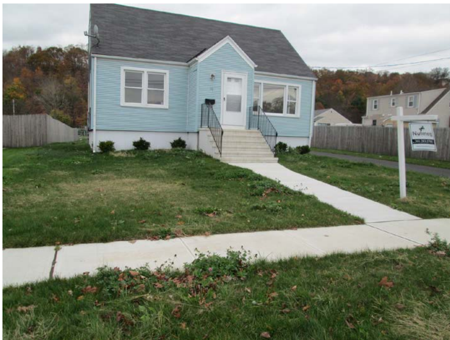
View looking northeast during the Fall 2012 inspection.
