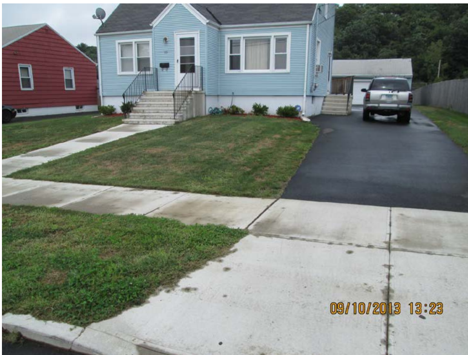
View looking northwest during the Fall 2013 inspection.
