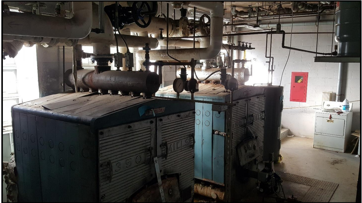
Building #3 Senn Building - Basement – Boiler Insulation (ACM)
