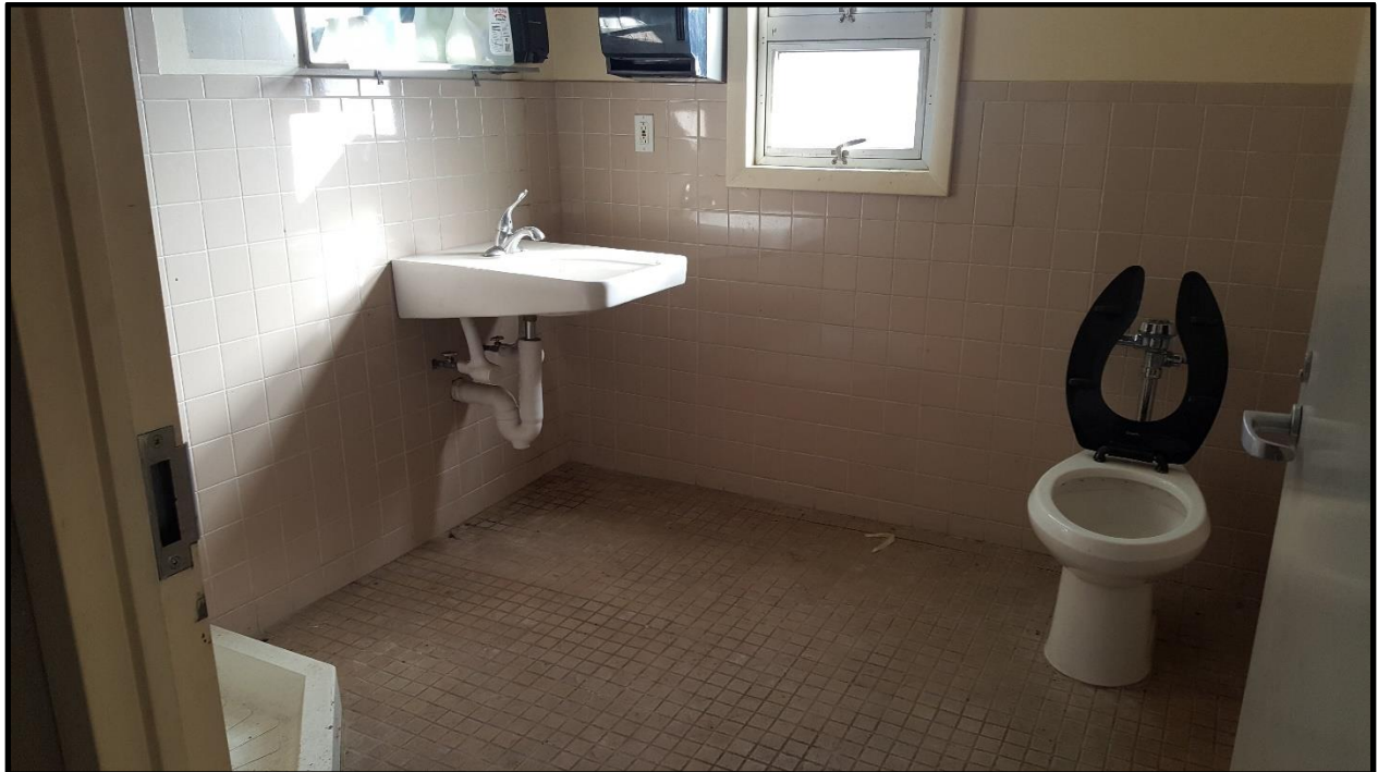
Building #9 – Maintenance/HVAC – Ceramic Tile Grout/Adhesive (ACM)
