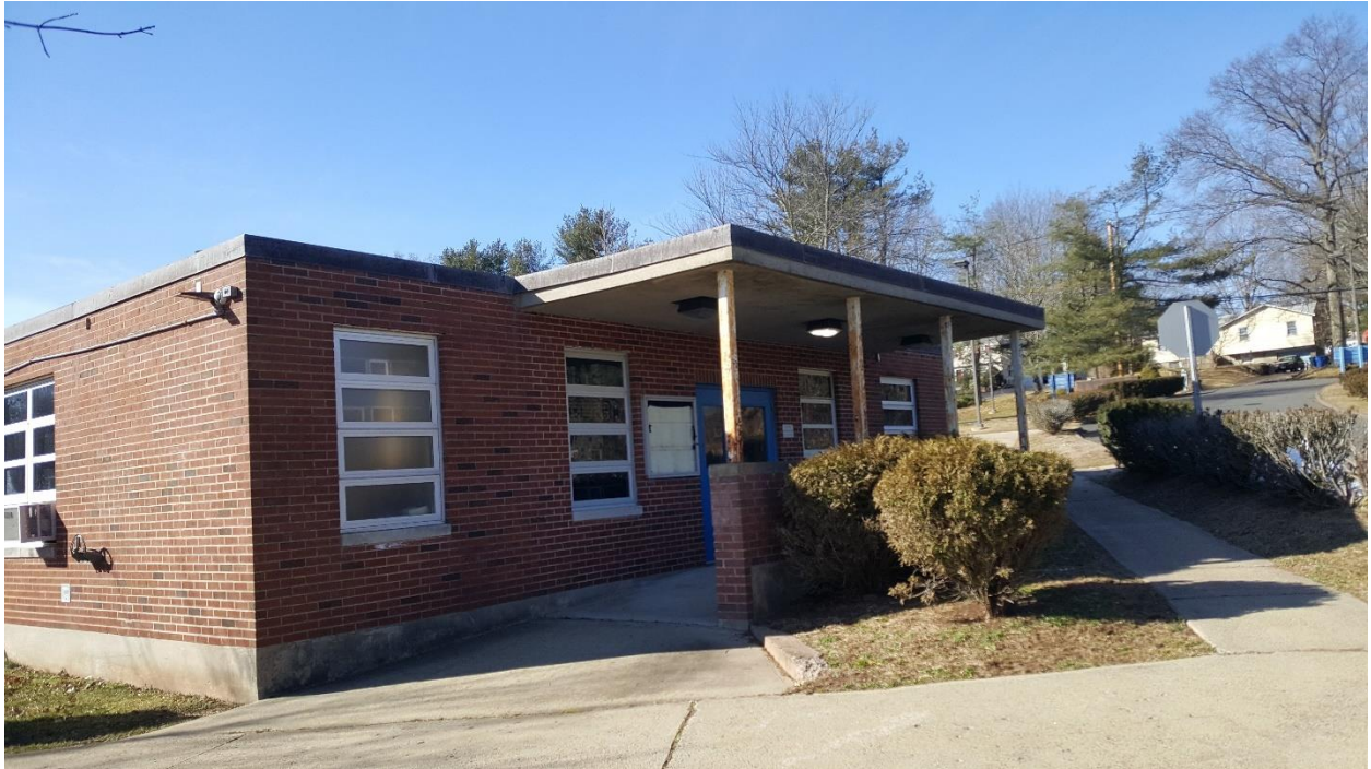
Building #3 Senn Building - Elevation – Window Caulk/Glazing, Blind Flashing (PACM/Suspect PCB)
