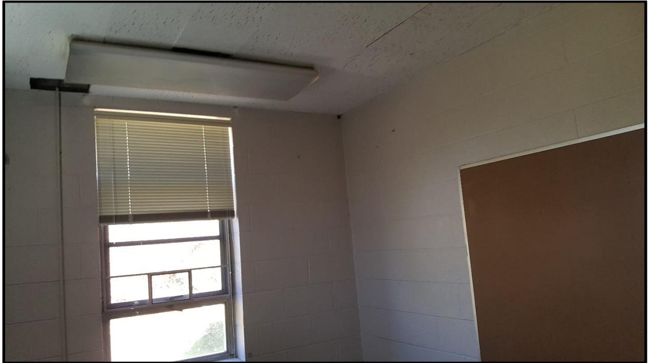
Building #5 Kitchen/Dining – First Floor – 1'x1' Ceiling Tile with Glue Daubs (ACM)
