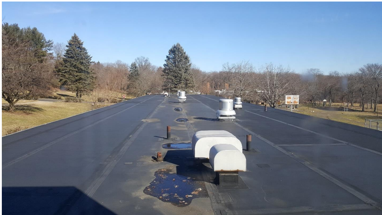
Building #3 Senn Building - Roof – Roofing (PACM)
