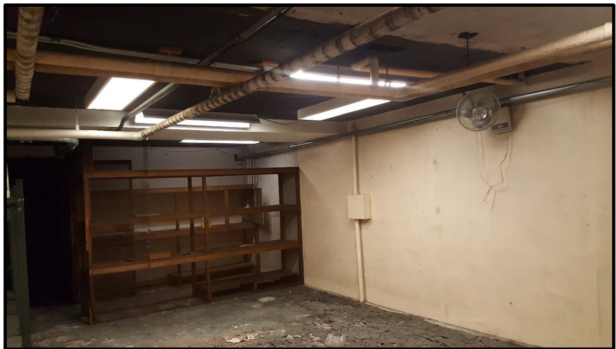
Building #5 Kitchen/Dining - Basement – Pipe Insulation (ACM & NonACM))
