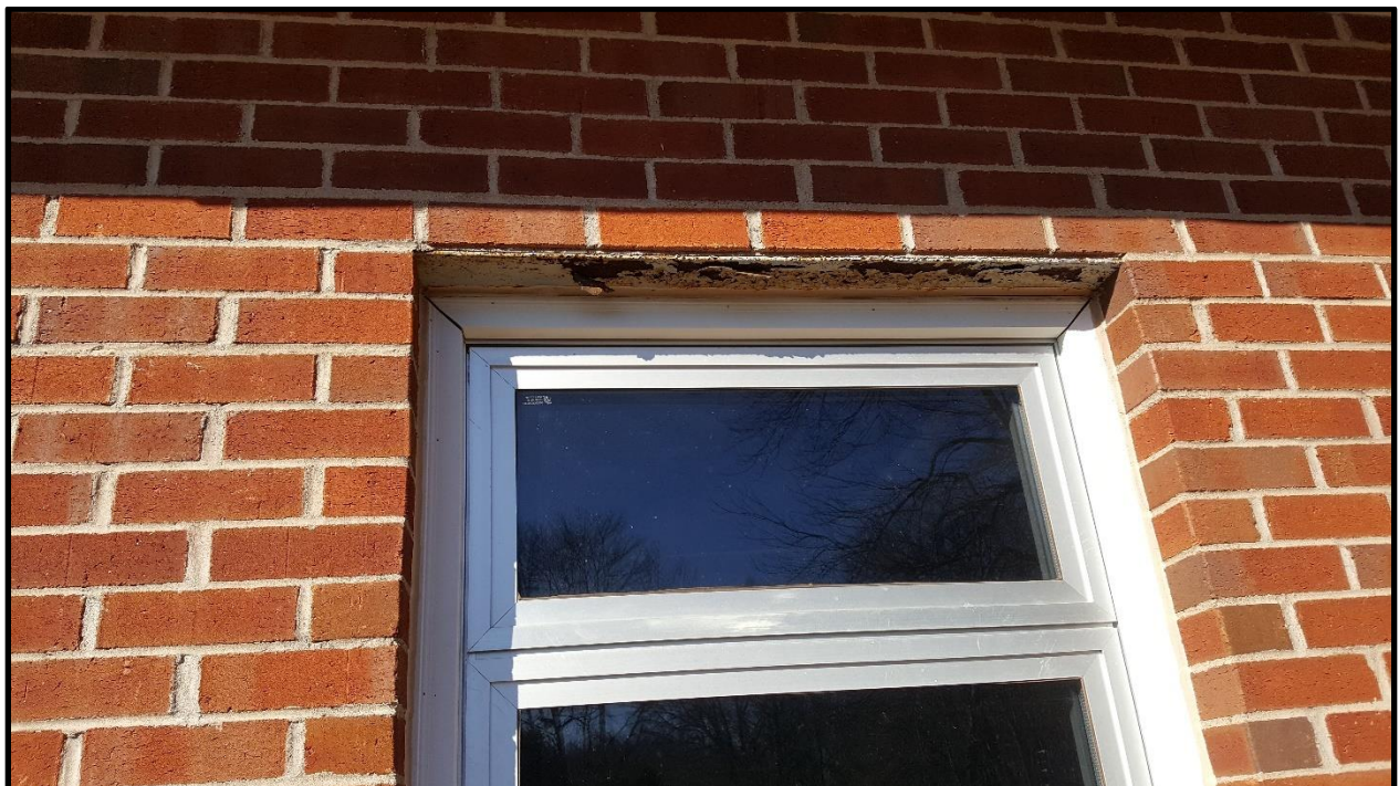
Building #9 – Maintenance/HVAC – Exterior Window Caulk (PACM/ Suspect PCB)
