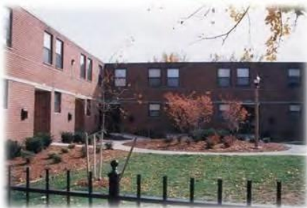
MLK Apts, Hartford, CT 64 Unit Rehab | $5.2 Million
