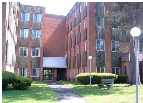
CT Scattered Sites 971 Unit Rehab $12.6 Million
