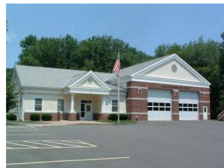
New Oakland Gardens Fire Station Farmington, CT $870,475
