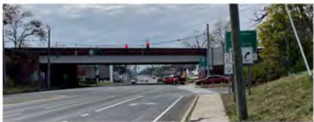
Figure 16 Dixwell Avenue at SB Route 15 Ramps – Skewed Crosswalk on West Side of Intersection
